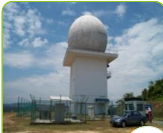
Weather Radar Stations
