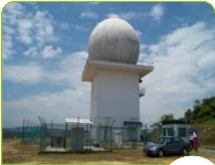
Weather Radar Stations
