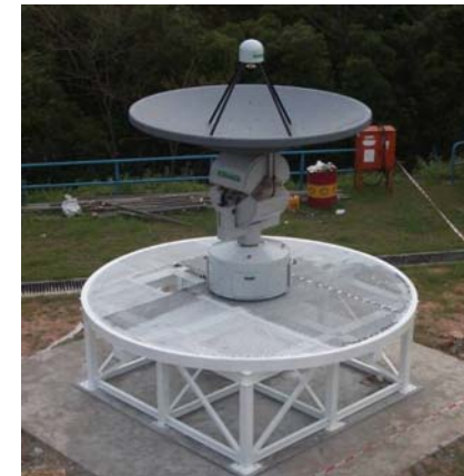
Tracking antenna for MODIS/POES at King's Park Met. Station
