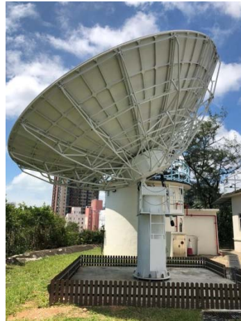
FY4 Satellite Reception System at King's Park Met. Station
