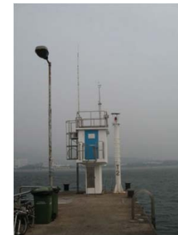
Tide gauge station
